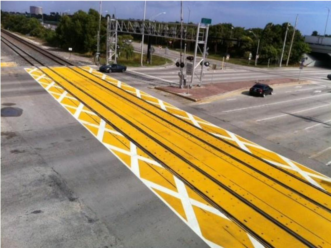
The federal Department of Transportation has tested the pavement marking and found some likelihood that it would increase safety, but felt that more field trials were necessary before they could reach a definitive conclusion.<sup>1</sup>
