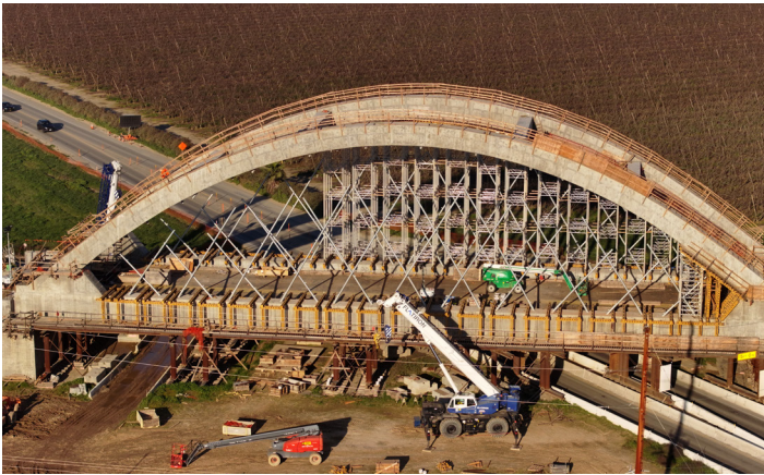
The Tied Arch Bridge in Fresno County will span 249 feet long and will take high-speed trains over State Route 43.
