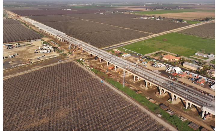
The Hanford Viaduct is the largest project in the 119 miles of construction. It spans more than 6,330 feet and will be home to the future Kings/Tulare Station.
