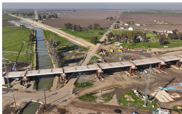
Corcoran Highway Grade Separation, Kings County, January 2026
