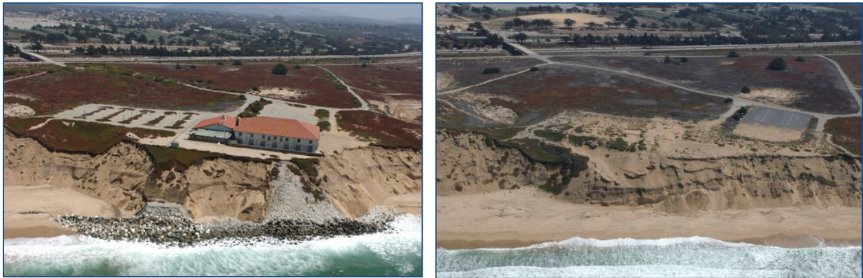
Figure 18. Photo depicting passive erosion. (Left) Passive erosion in front of a revetment at Fort Ord, illustrating the loss of beach where the development prevents the shoreline from migrating landward. The beach continues to migrate inland on either side of the revetment. (Right) Recovery of the beach following removal of the revetment and blufftop structure. (Source: California Coastal Records Project ).
