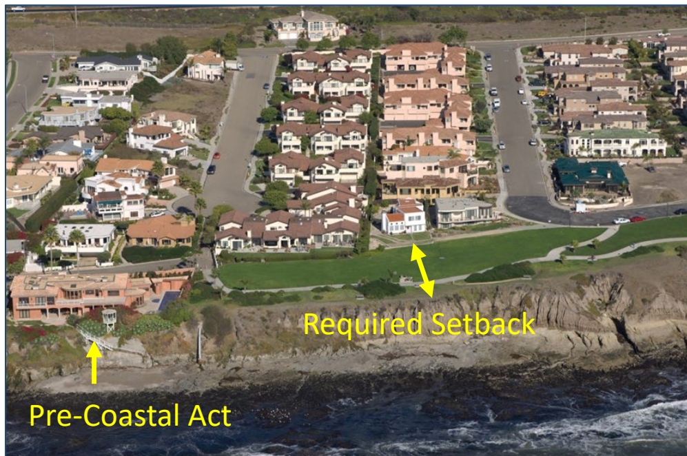
Figure 21. Photo depicting a development setback in Pismo Beach. (Source: California Coastal Records Project )
